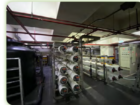
The second stage of wastewater recycling and reuse equipment in OSE Central 3rd Factory (HQ)
